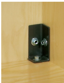
Two, triple-bolted corners for extra strength
